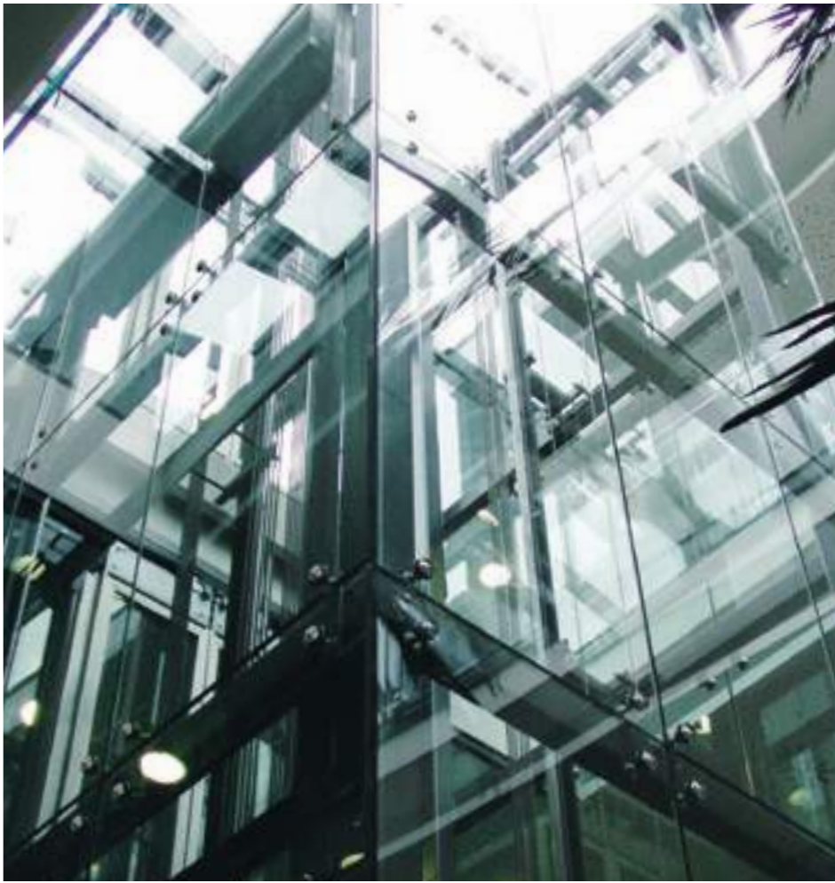
Tubular hoist frame, square tube Point mount glass fixing, Glazing in front of the profiles
