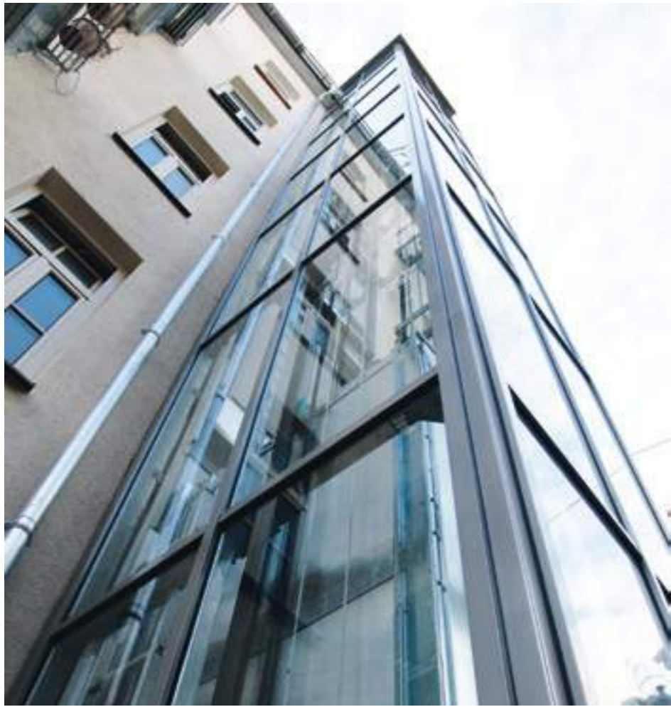
Tubular hoist frame, square tube Aluminium façade profile
