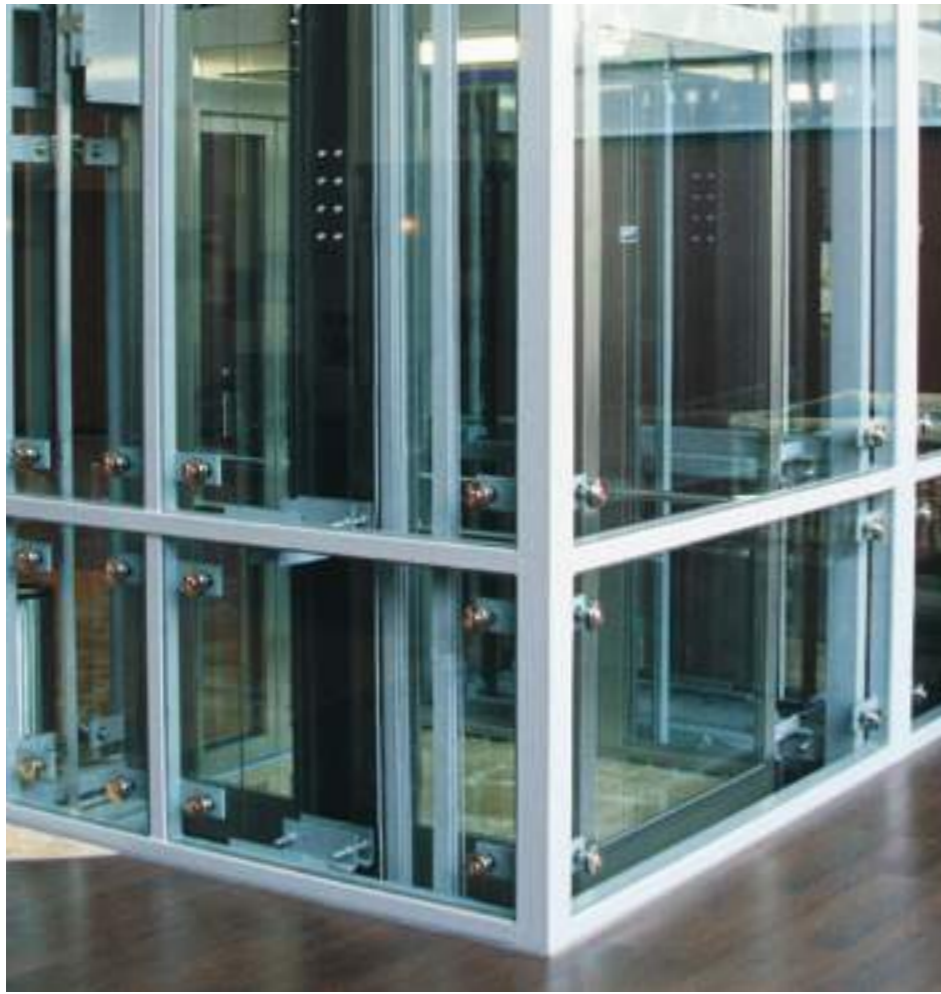
Tubular hoist frame, square tube Point mount glass fixing, Glazing between the profiles
