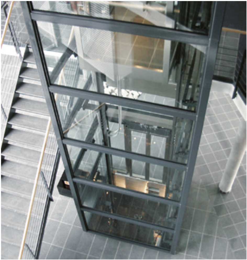
Tubular hoist frame, square tube Glazing between the profiles
