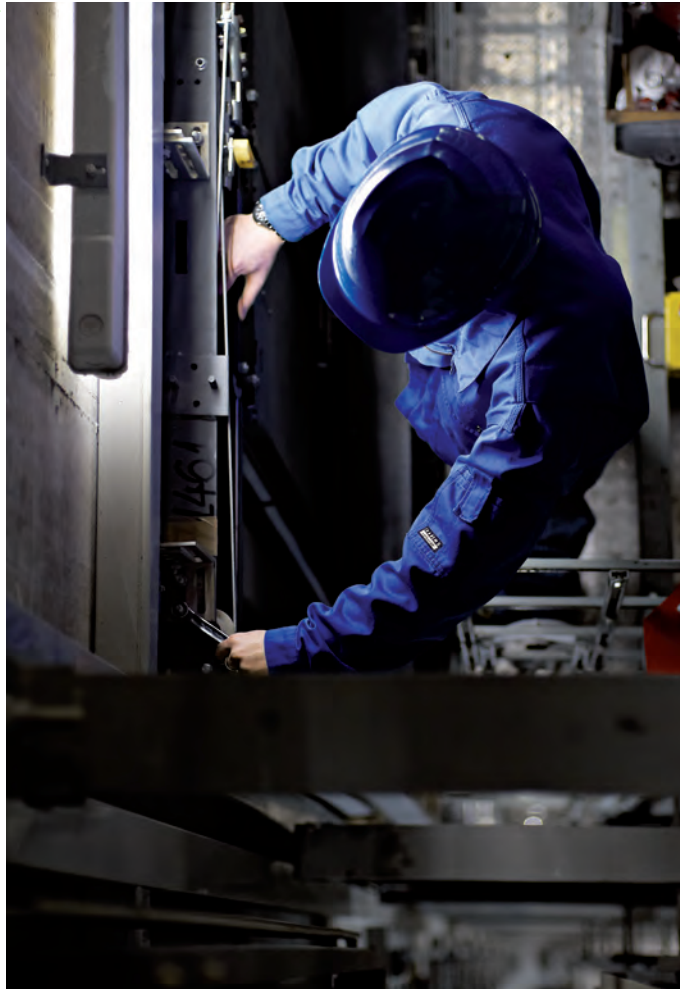
4 Setting work on the shaft door
